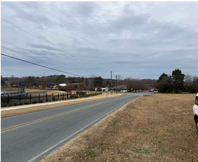
Looking N on Plyer Rd
